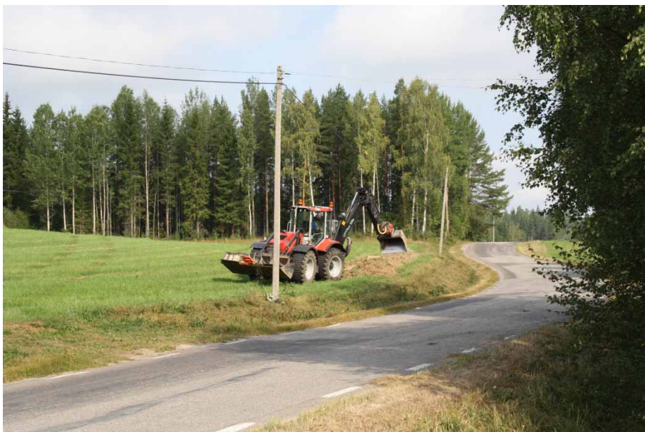
Figur 8. Schakt 3. Foto: Anders Altner.
